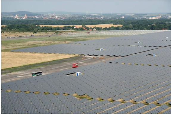
Waldpolenz Solar Park, Germany
