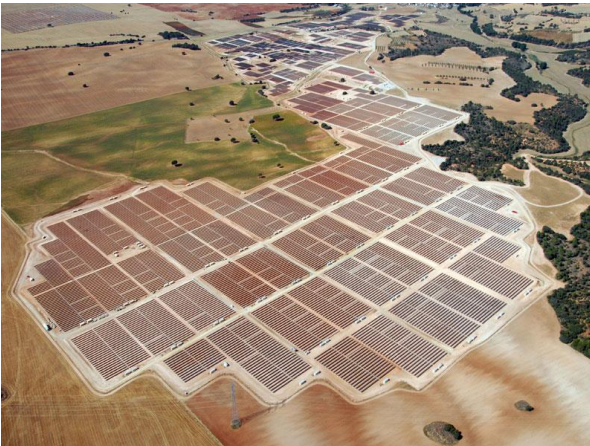
Olmedilla Photovoltaic Park, Spain
