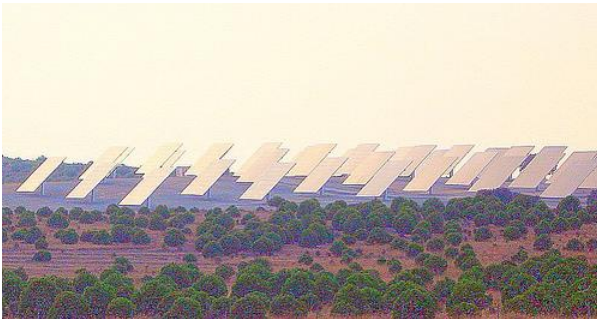
Moura photovoltaic power station, Portugal
