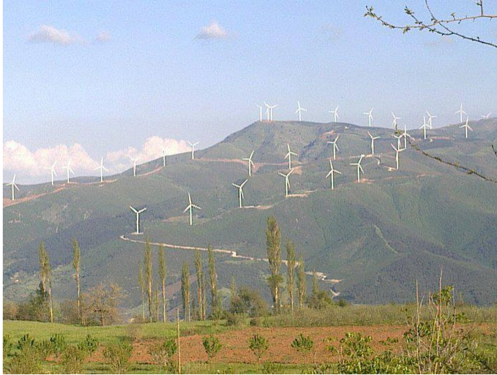
Osmaniye-Bahçe 135 MW wind power plant
